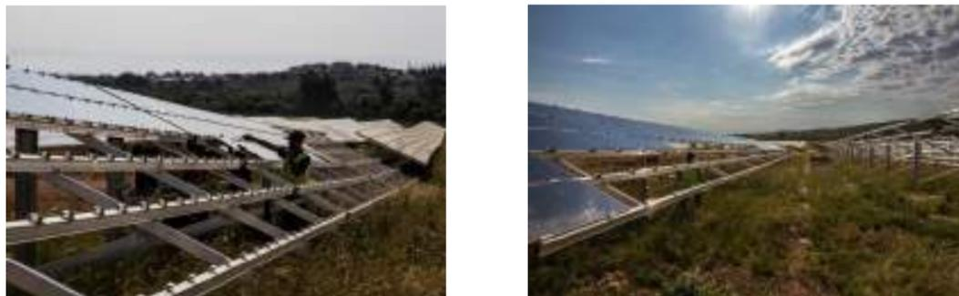
Figure 12. Montage des structures supports (source : NEOEN)
